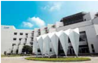
Tainan Plant (Diamond-rated Green Building)
